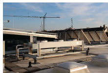
Recooling unit (roof)
