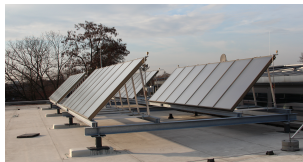
Plate collectors (roof)
