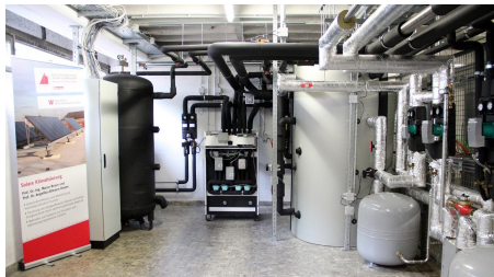
Control cabinet, cold storage, ACM, hot storage, pumps (cellar)
