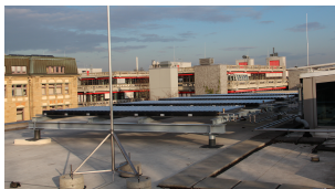
Vacuum tube collectors (roof)
